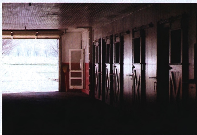
State of the art ventilation is built into the design for barn renovations, which are well underway (top). The broodmare barns will retain catwalks above the stalls. Yearling barn (above) in current use is typical of the old style, with low tongue-and-groove ceilings. The small windows at the back of each stall were removed to accommodate Dutch doors for ventilation. Stall doors will be open screen work like that typically seen in modern barns.
