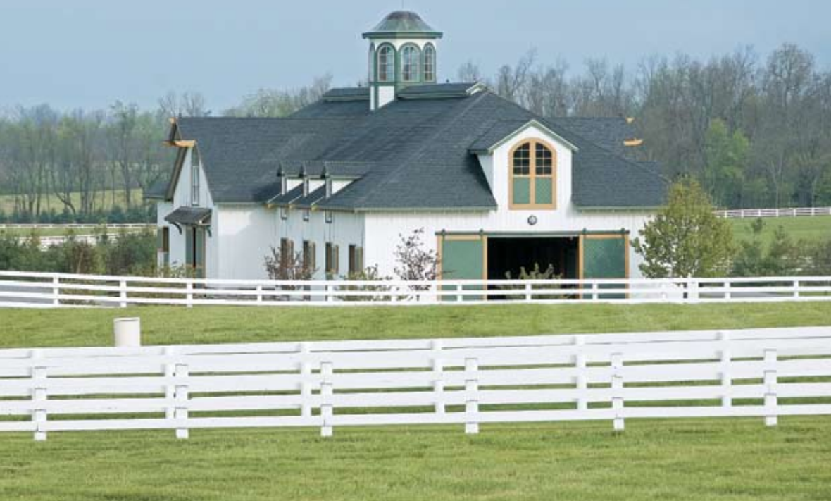
Top, John Blackburn has designed horse barns all over the country. Above, unlike old-style barns that were often built with haylofts, making them dark and cave-like inside, the Monticule barns have 32-foot open ceilings and large dormer windows dropped down to let more light into the stalls. Their design includes an innovative airflow pattern with cross ventilation and vertical ventilation.
