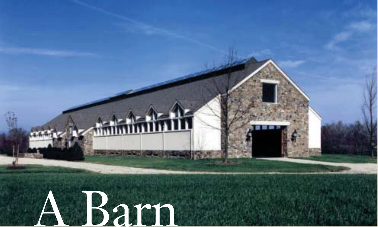
Courtesy Blackburn Architects (2)
