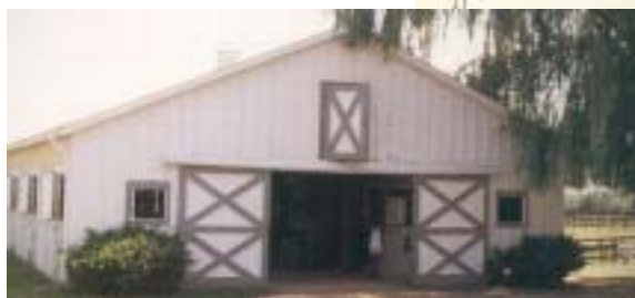
Inset: Moderate in size, this six-horse show barn includes a wash stall, kitchenette and could be designed with upgrades, such as a bathroom, aisle ceiling, etc.
