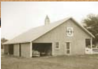
This four-stall barn with run-in shed under the same roof allows the owner to save money on materials. The corners are edged with metal stripping to prevent damage from cribbing horses that may be turned out for the run-in shed function.
